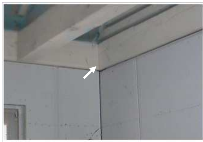
Figure 17 South East Top Corner – Visible
