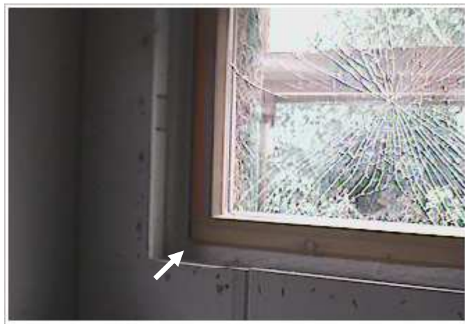
Figure 22 East Windows North Corner – Visible
