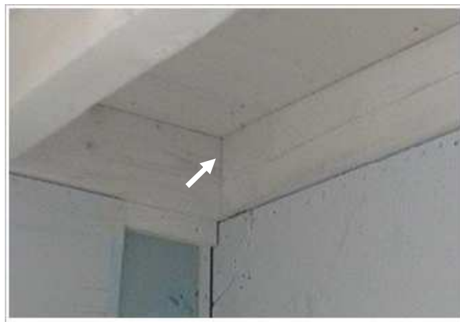
Figure 19 Southwest Top Corner – Visible
