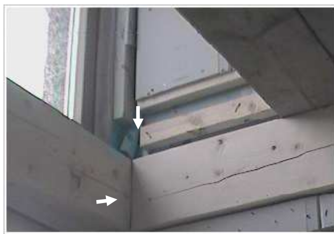
Figure 8 South West Corner Living Area – Visible
