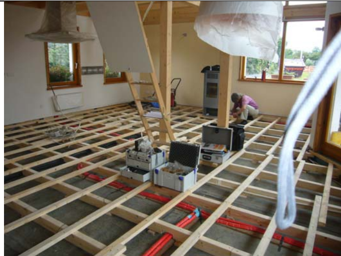
Picture 1: VOC adsorption in the house's living room during reconstruction work
