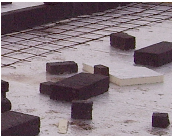
“Funny”! – Some builder make the last screed before walls & roof – a wet floor for years and mould later on is no problem – they said! Auah!
