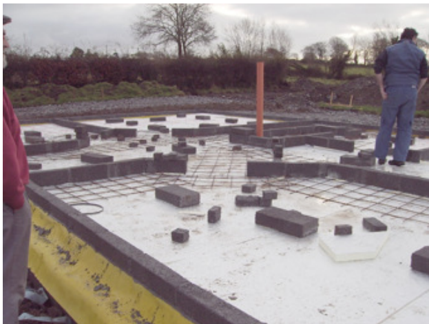
“Funny”! – Some builder make the last screed before walls & roof – a wet floor for years and mould later on is no problem – they said! Auah!
